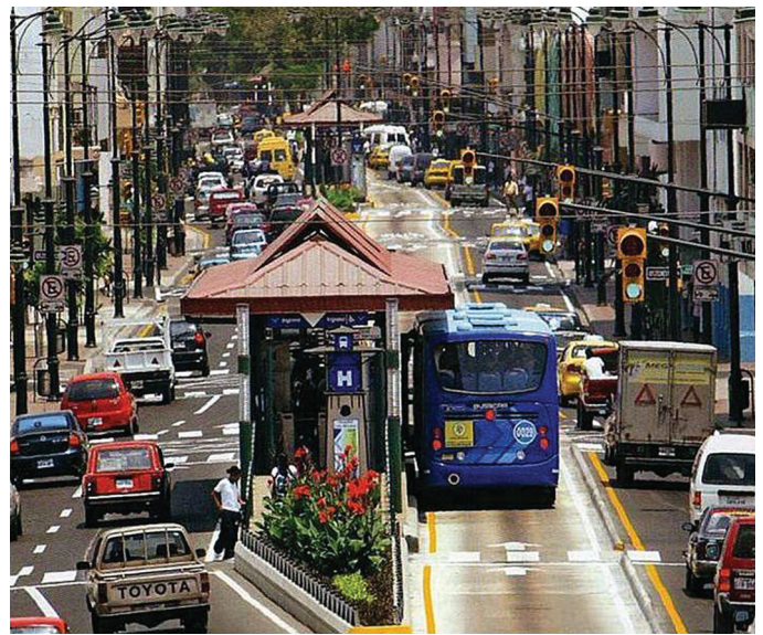
A dedicated one-directional BRT lane in the middle of a one-way street in Guayaquil, Ecuador. Photo: ITDP
