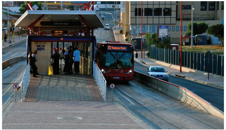
An example of Johannesburg's Rea Vaya BRT lane in the central verge of the road. Photo: ITDP
